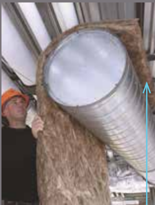
Fiber glass is used in commercial buildings, as well as can be found insulating pipes and ductwork.
