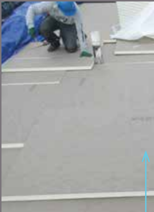
Closed-cell foam insulations, like polyisocyanurate (shown here with organic facers), combine traffic and moisture resistance.
