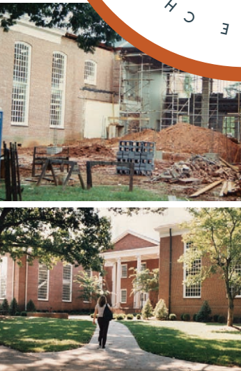
1993 Ethel K. Smith Library renovation began (top) - completed 1995 (bottom)
