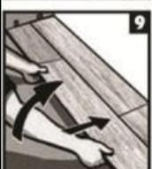
**Figure 9:** Continue step 8 system on the remaining planks in the row. At the end of the row repeat steps 4, 5 and 6.
