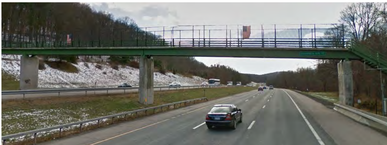
Top, left to right: Platform at Harriman Train Station; Exit 16 Harriman Sign on the NYS Thruway Bottom: Southfields pedestrian bridge across I-87
