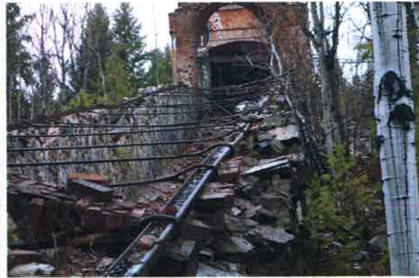
Detail of the exposed Flume tensioned cables.
