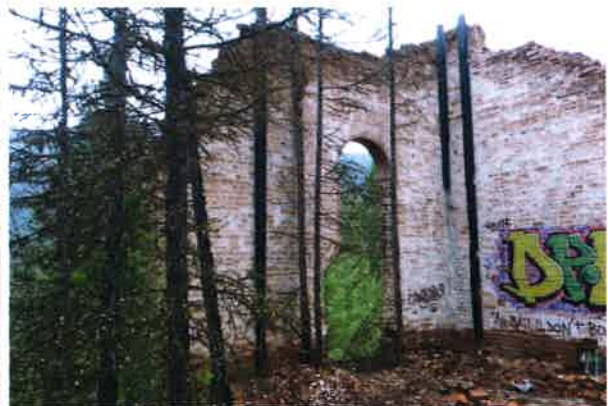
Corner Building walls.
