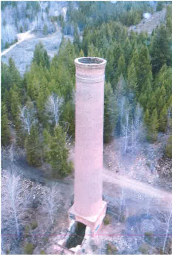
Aerial view of the Chimney and collapsed flume.
