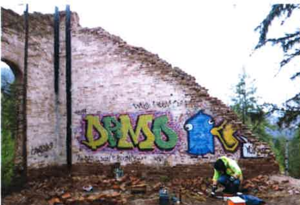
Corner Building walls.
