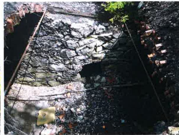
Flume tensioned cables and rock block wall.
