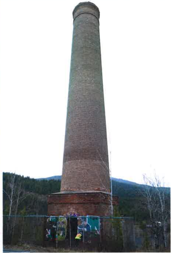
Chimney view from access road.
