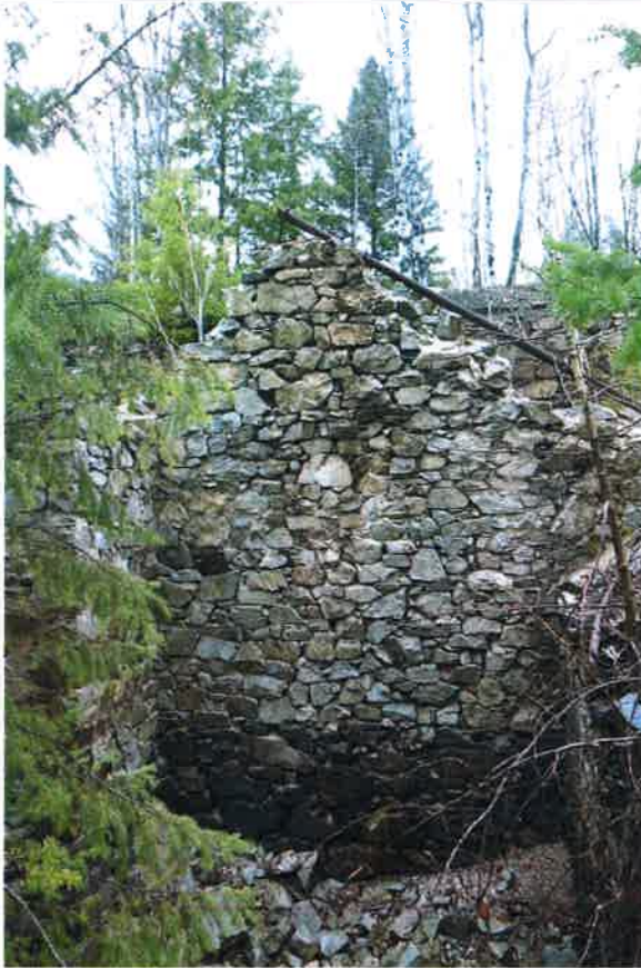
Rock masonry wall of the smelter complex.
