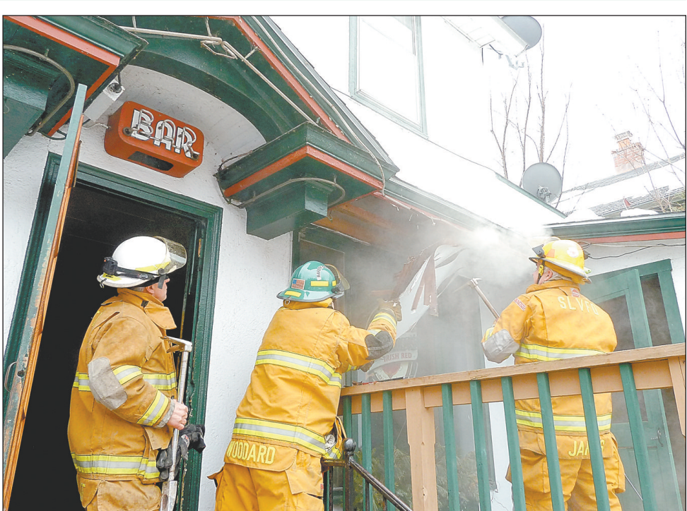
Smoke pours out as Saranac Lake firefighter Vernon James uses a crowbar to rip open the eaves of the Belvedere Restaurant early Tuesday afternoon to extinguish a fire smoldering in the front wall of the bar. (Enterprise photo — Peter Crowley)
