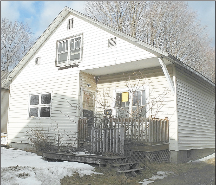
Village of Tupper Lake officials have declared that this house at 10 Front St., co-owned by Natalie Frank of Tupper Lake and Mark Keating of Schenectady, is unsafe and must come down.
