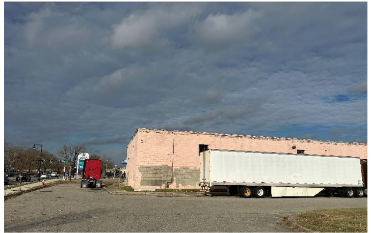
Existing conditions west of the warehouse building. Looking north from South Water Street.
