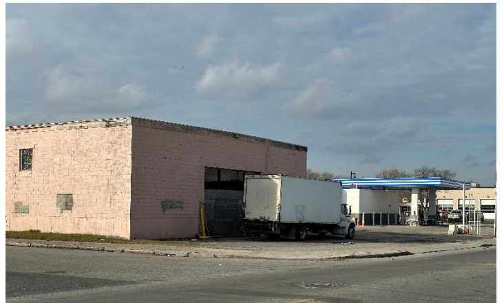
Existing site conditions east of the warehouse building. Looking northwest from South Front Street.
