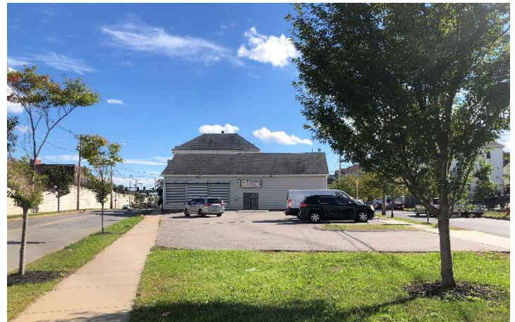
Parking lot and front of building. Looking south from northerly property boundary.
