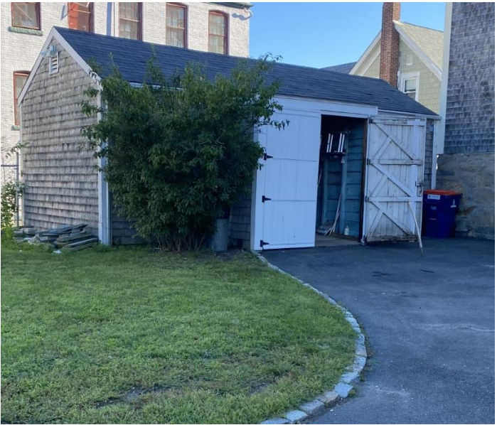
Existing South Façade and hardscape
