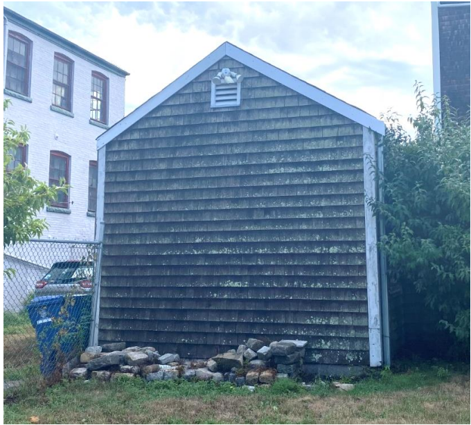
Existing West Facade
