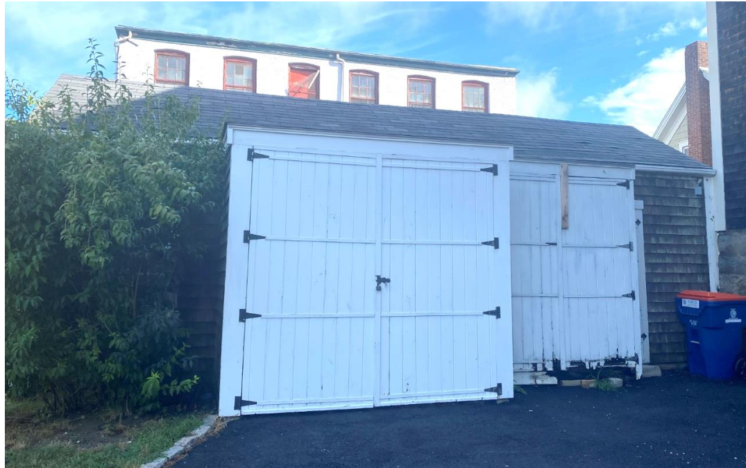
Existing South Façade- Entrance bump out to be removed and doors replaced.
