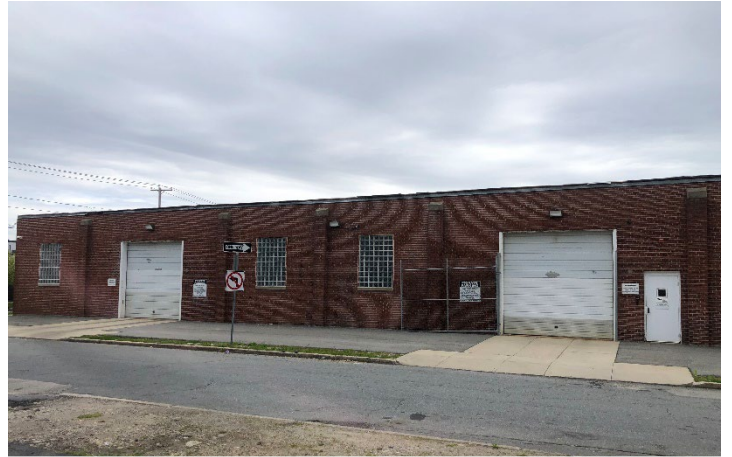
Overhead doors at rear of building. Looking east from abutting parking lot across Jenney Street.
