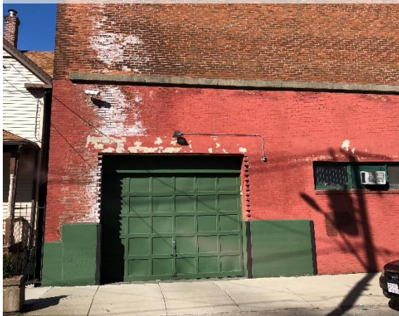
Southeast overhead door to remain. Looking west from Jean Street.
