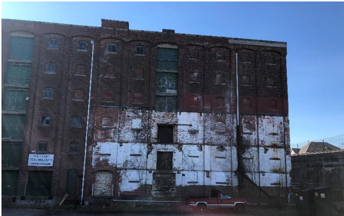
North façade to be stripped to brick, proposed canopy area. Looking south from northwest area of site.
