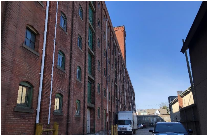
North façade with existing leaders, fire service to remain. Looking west from Jean Street driveway.
