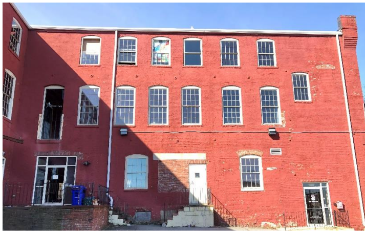
East-facing façade stairs to be removed, lighting to remain. Looking west from parking lot.
