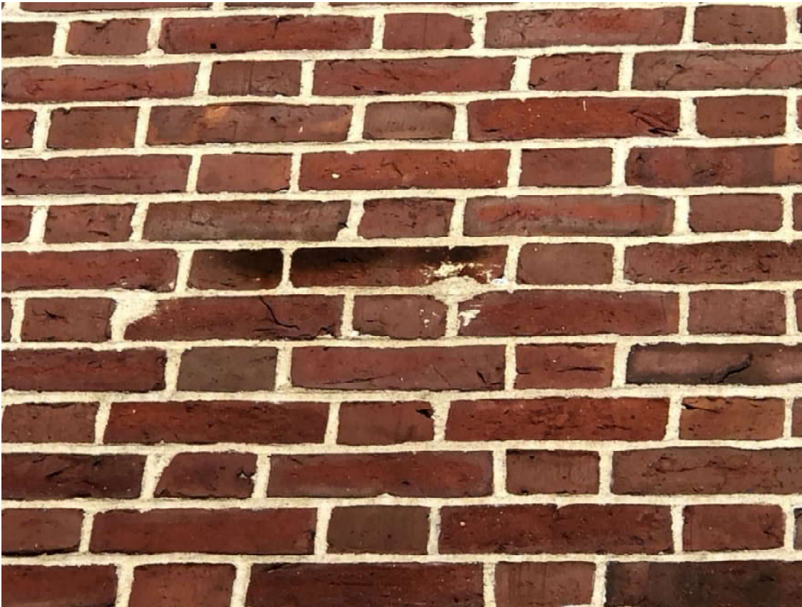
5. Bourne Building, South Elevation, deteriorated mortar, cracked, spalled brick
