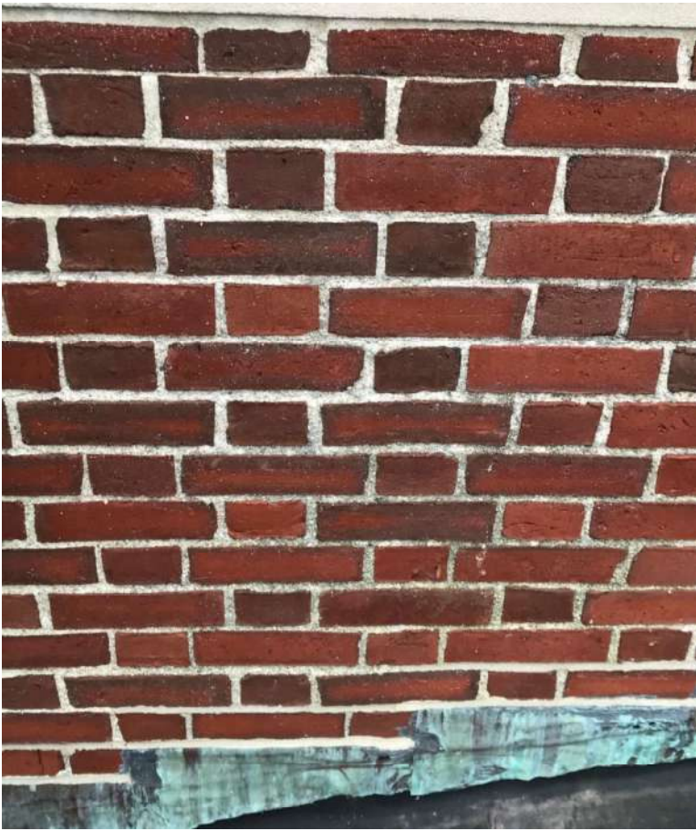
7. Bourne Building, North Elevation, deteriorated mortar, cracked, spalled brick
