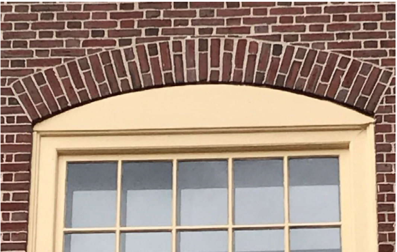
6. Bourne Building, South Elevation, backer rod needed to address gap at lintel
