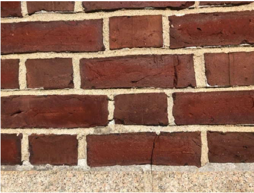
3. Bourne Building, West Elevation, deteriorated mortar, cracked, spalled brick
