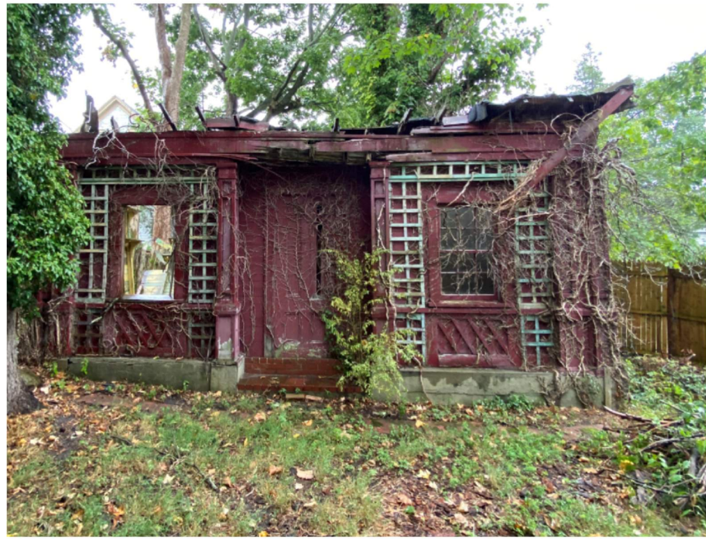
EXISTING STRUCTURE PHOTOS - WOOD FRAMED "TEA HOUSE" ON CONCRETE SLAB
