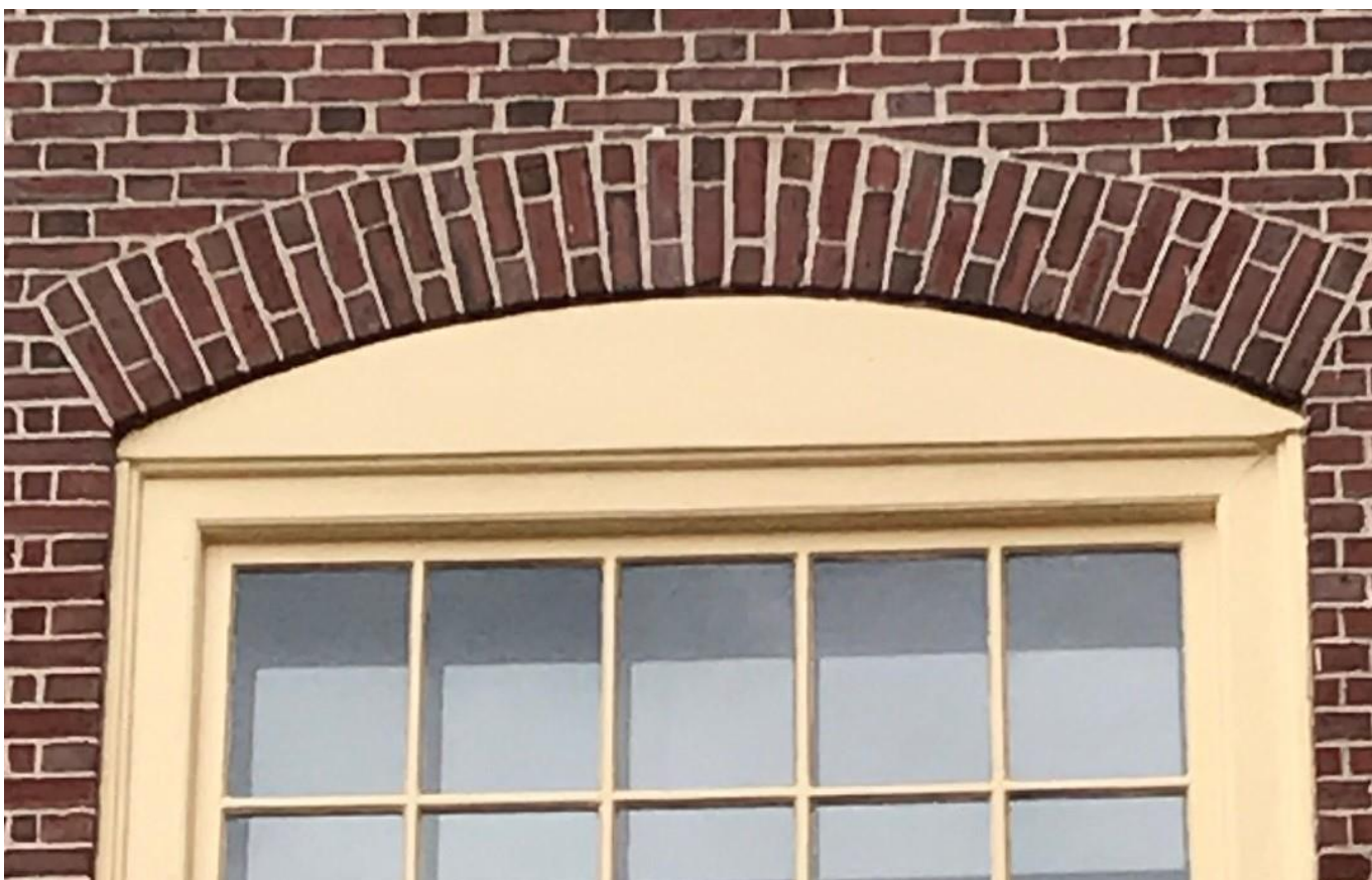
12. Bourne Building, South Elevation, backer rod needed to address gap at lintel
