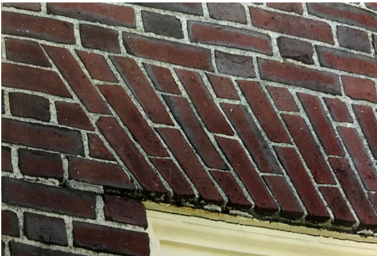
5. Wood Building, North Elevation, failing angle iron lintel
