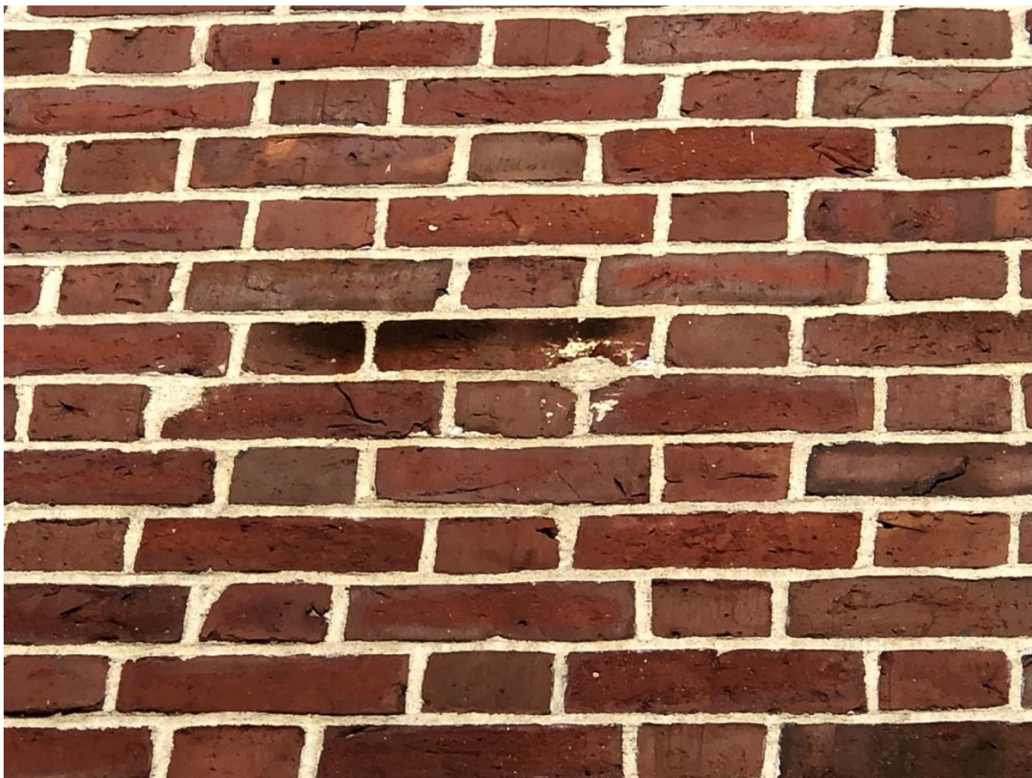
11. Bourne Building, South Elevation, deteriorated mortar, cracked, spalled brick
