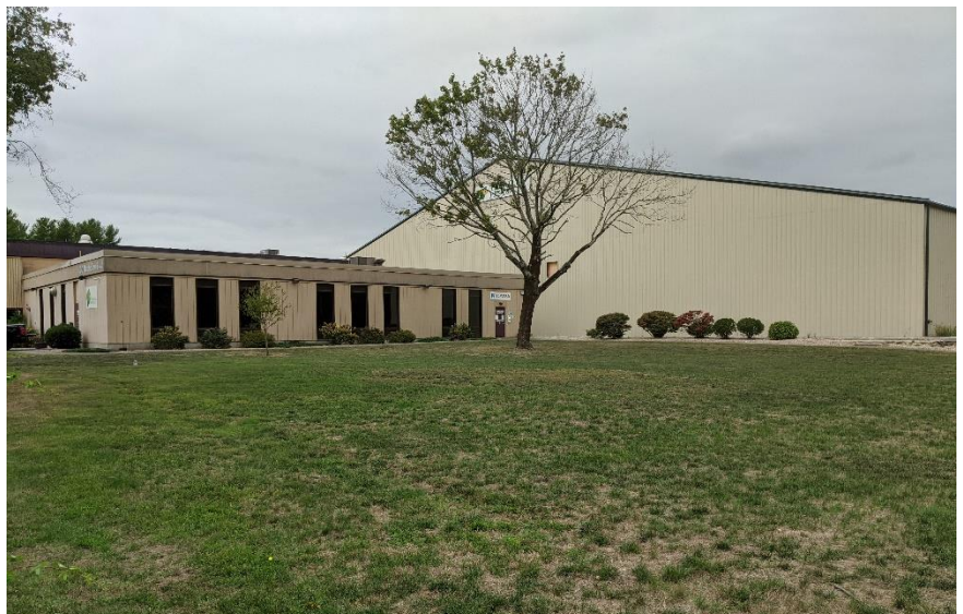
Southeast corner of the building complex Looking northwest from internal roadway
