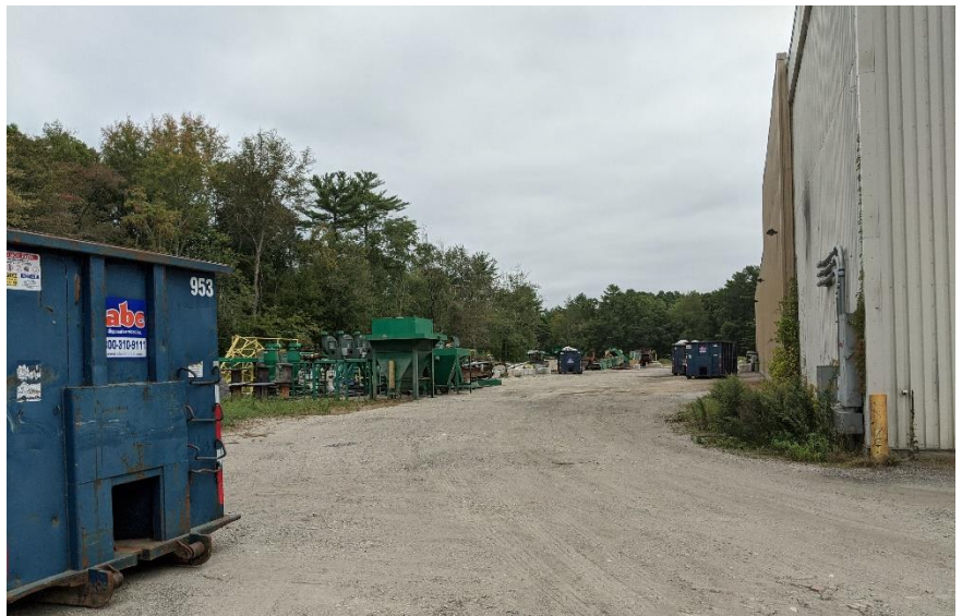
Location for proposed solar array/rail line depot Rear/North Elevation- looking east from northwest corner of building/site
