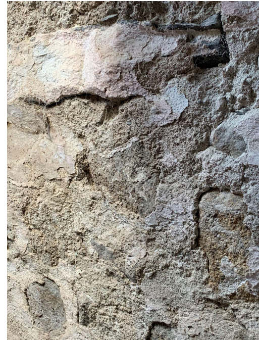
20. Crack in foundation.
