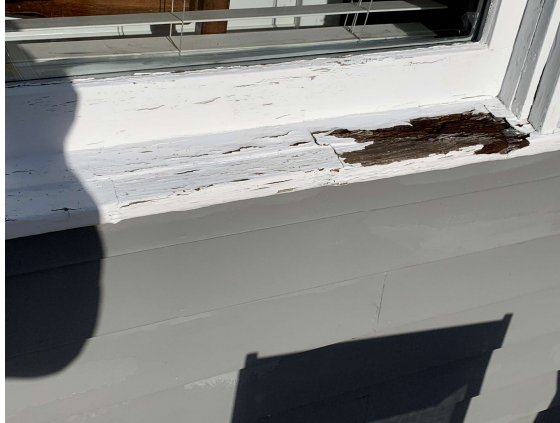
5. Front window showing water and rot damage.
