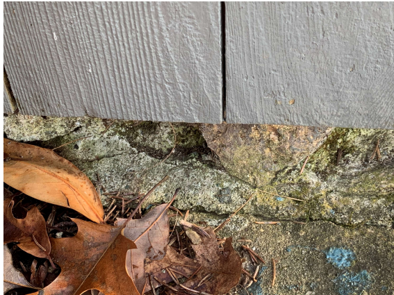
4. Cracks in rock foundation which would need to be repaired. Structural integrity is in question.
