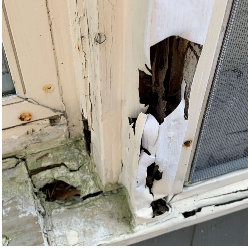
10. Bedroom window rot and water damage.
