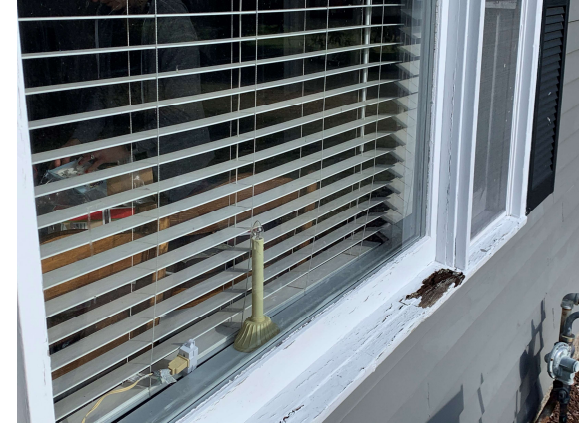
6. Continuation of rot damage of front window.
