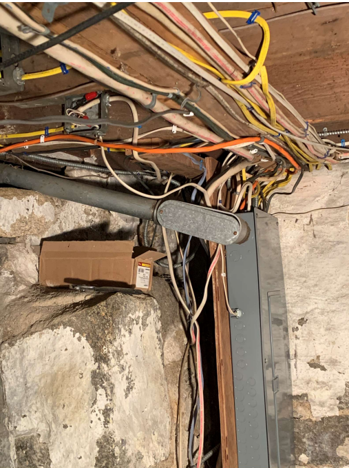
12. Electrical would need to be completely removed and rewired.
