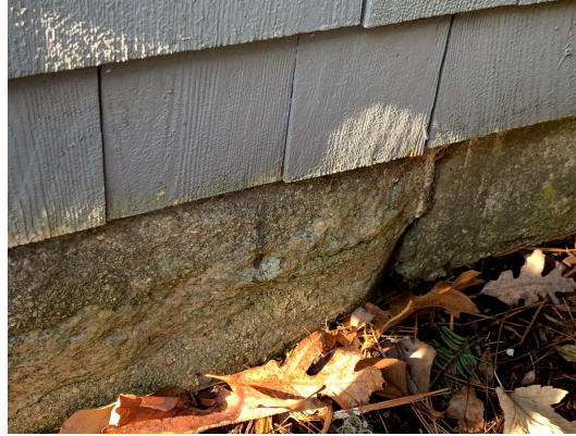
8. Cracks in foundation.
