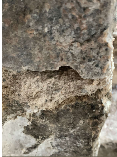
11. Crack in foundation.
