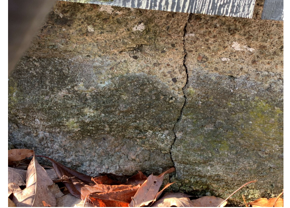
9. Crack in foundation.
