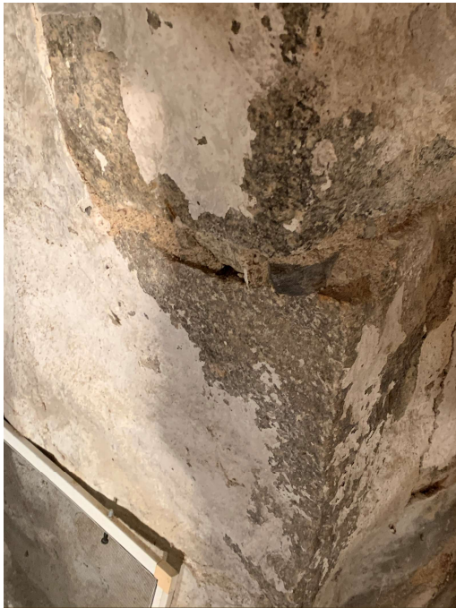
15. Crack in foundation.
