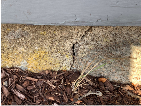
7. Cracks in foundation.
