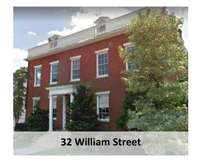
**OVERVIEW:** The applicant is seeking to rehabilitate the building performing work to the following items: Replace gutter, downspouts and soffits; repair and paint roof balustrade; repair/replace dormer window sashes; repoint exterior brick masonry.
