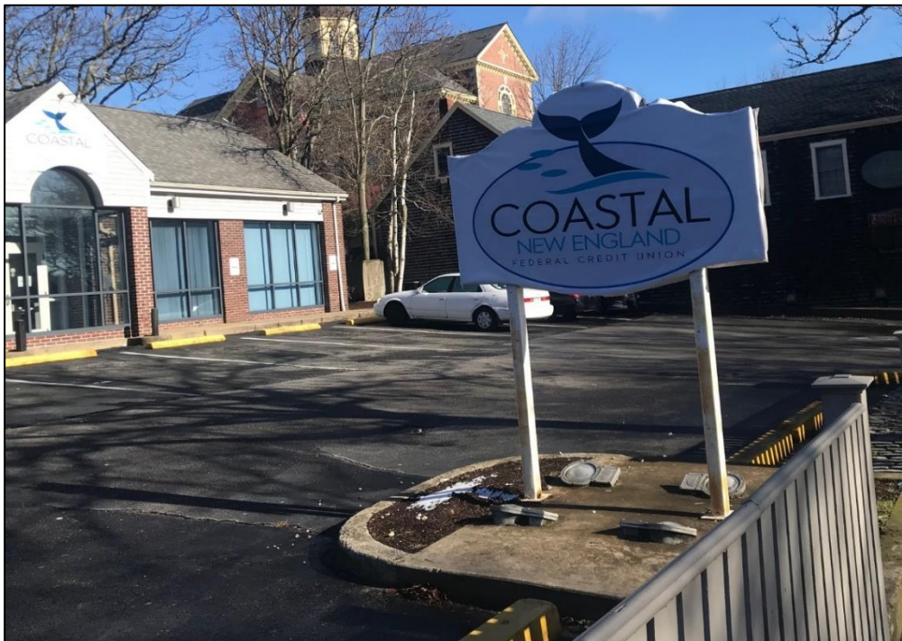
CURRENT EXISTING CONDITIONS- Double-faced post sign and wall sign with temporary banner wrap.
