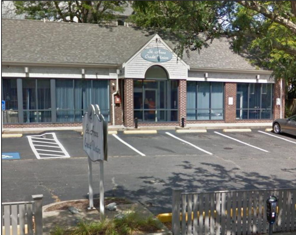
PRE-EXISTING CONDITIONS- Double-faced post sign and wall sign
