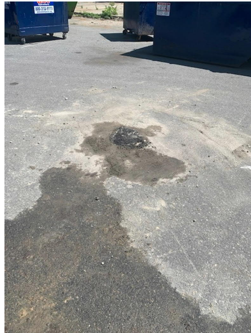
Figure 2: Example of backfilled borehole
