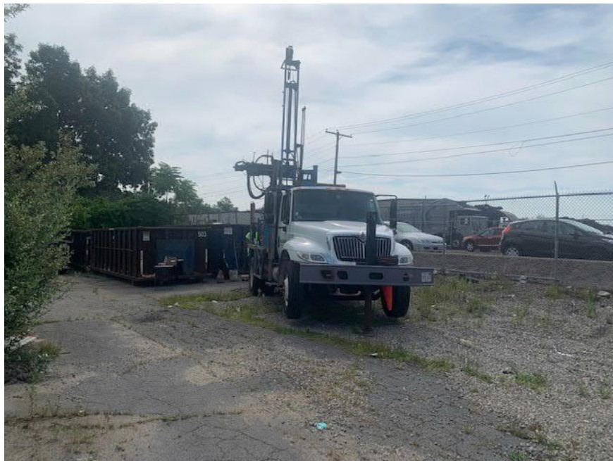
Figure 6: Drill rig setup at P-33
