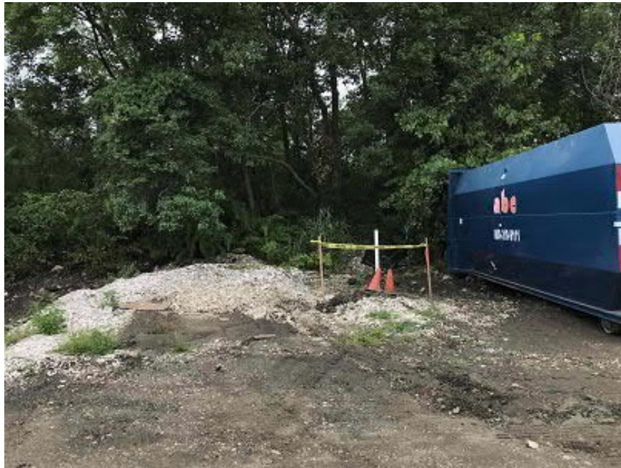
Figure 5: Installed monitoring well
