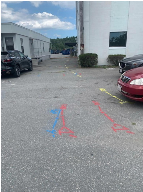
Figure 1: Utility mark-out
