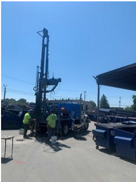
Figure 3: Drill rig setup at P-22
