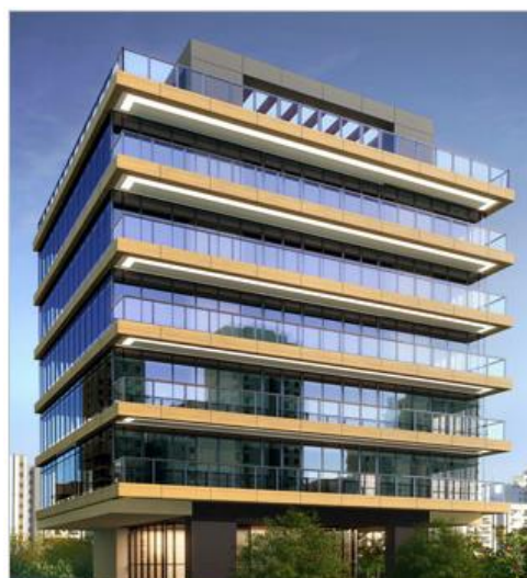
Casa do Ator Office Building in SP Update: Sale of the entire building
