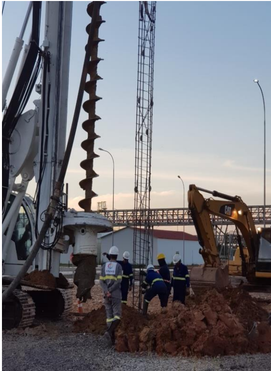
Execution of stake of boiler 32
