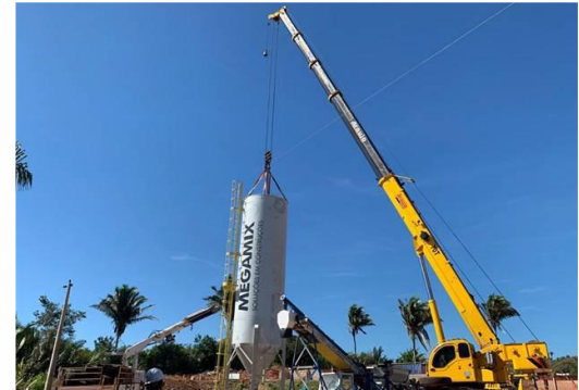
Concrete plant installation
