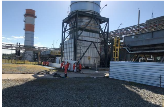
Installation of operational siding
