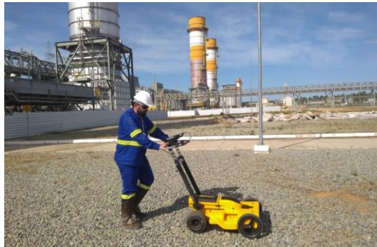
Execution of soil scanning activities
