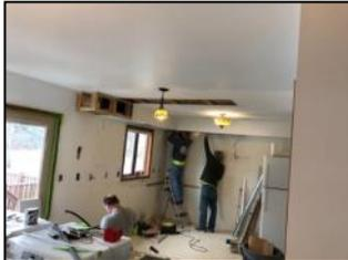
All of the old cabinets, countertops and oak backsplashes were removed from the kitchen. Brian Elder and his team spent a full day and two partial days removing and repositioning the soffit, sheet rocking and spackling, and installing a vent for the new stove fan (the old one recirculated air back into the kitchen and Jeff said it would regularly set off the smoke alarm).
