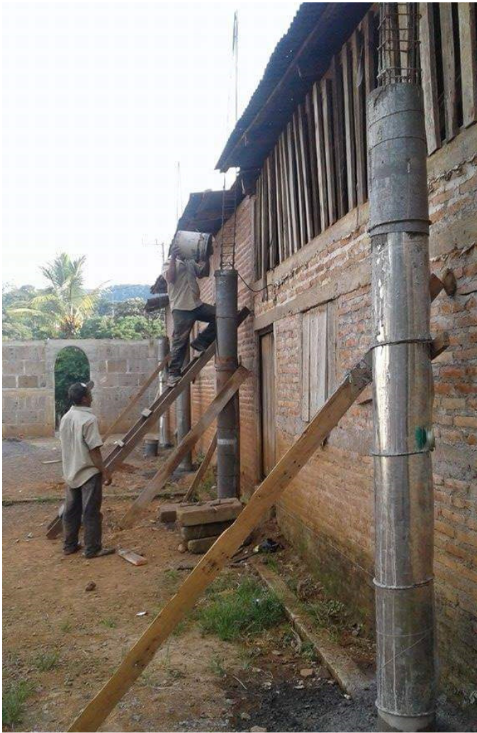
The columns go up to the roof line and will help support the new wall as well as the 2x4 rafters to which tin will be added to complete the roof.
