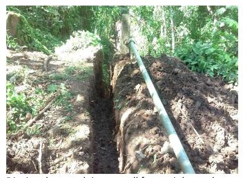
Digging the trench is no small feat as it has to be dug by hand. At this time water that is not contaminated with strychnine has to be carried from a long distance. This pipeline will give the village easier access to clean water.
