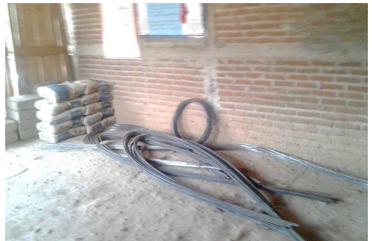
This wall is to a small room where the church meets now and they are showing the re-bar and cement purchased with money we have sent to help build a sanctuary and class room.
