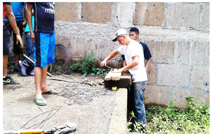
After church they went out to work on their new building. Here a man bends re-bar for footings and wall support.
