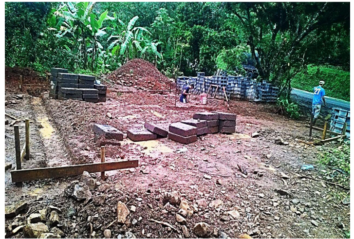
Starting the construction of the Medical Center, that will be staffed by a doctor, two nurses, and an ambulance.
