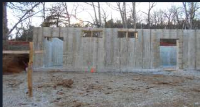
New Camp Showerhouse!
