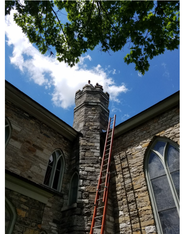
Maintenance work begins on the turret.
