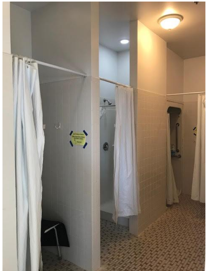
Example of showers (women's room in photo)
