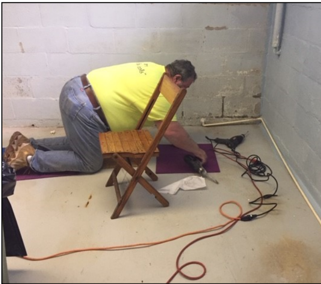
Spencer is drilling holes to put a drainage system in. Hopefully this addition will stop any water coming in after a rain and release pressure on that wall.
