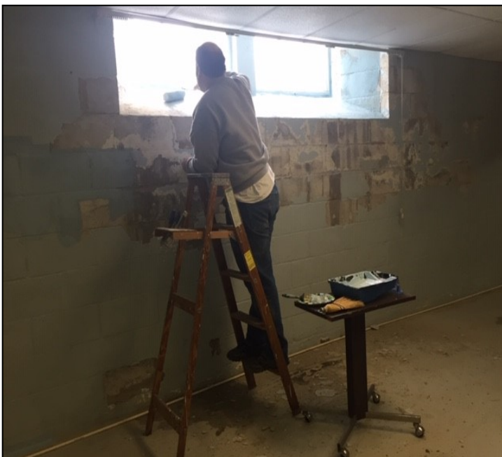
Spencer is drilling holes to put a drainage system in. Hopefully this addition will stop any water coming in after a rain and release pressure on that wall.
