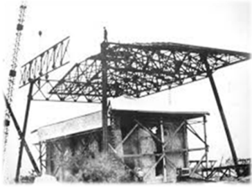
Construction of the second roof over Casa Grande Ruins
