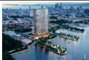
36-story 620 unit residential tower at Wharton Piers is slated to break ground in 2027
