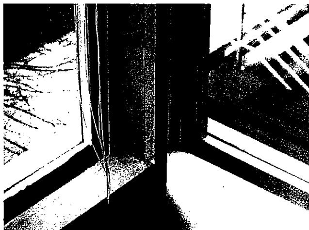
5. Corner of windows - Apartment 306
