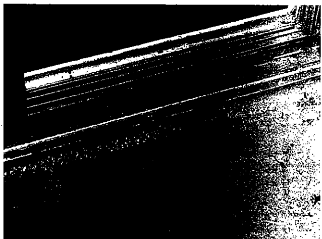
6. Balcony membrane termination at door sill
