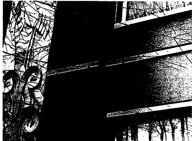
2. Cross-cavity flashing
