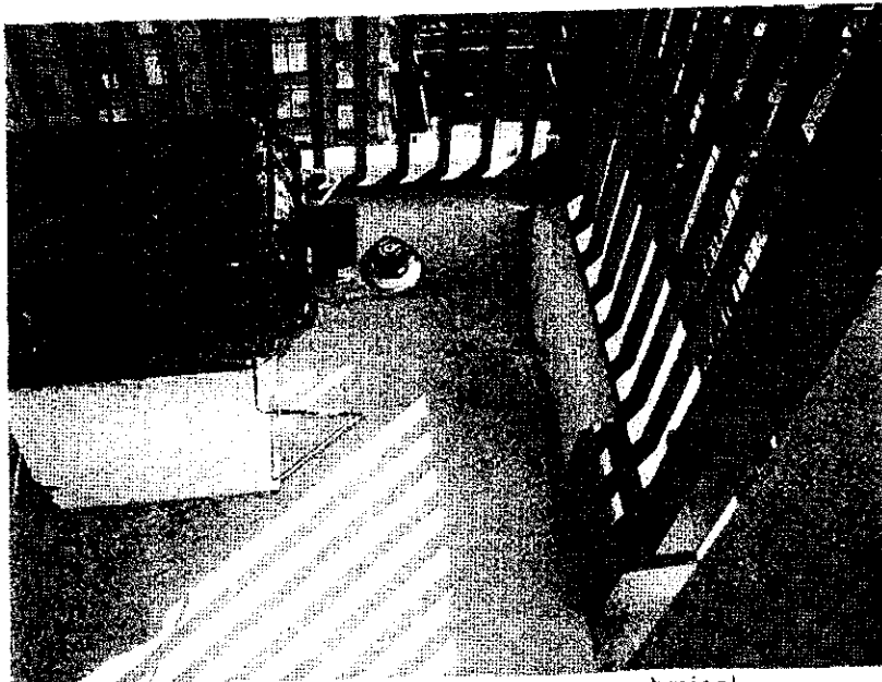
Photo 4: Dirty balcony membrane- typical.
