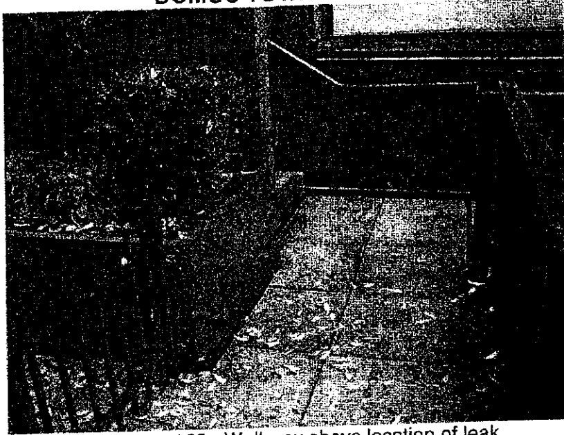
Photo 07 1063: Walkway above location of leak.
