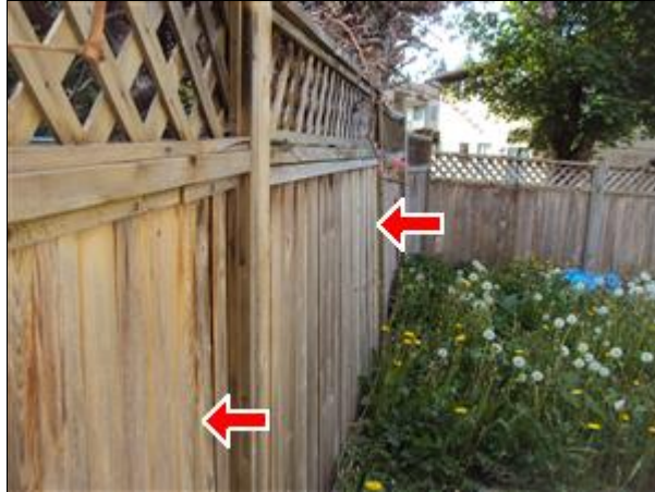
2.6 Picture 2 Perimeter Fencing
