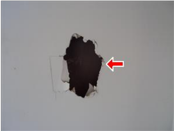
4.1 Picture 2 Interior Walls
