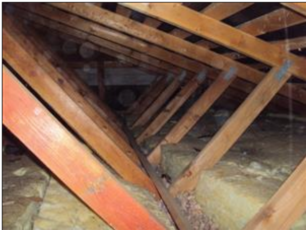
5.5 Picture 1 Engineered Wooden Trusses
