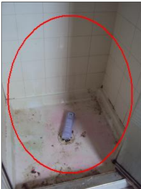
6.1 Picture 3 Clean & Seal Grout
