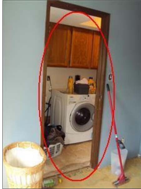
4.5 Picture 2 Missing Door
