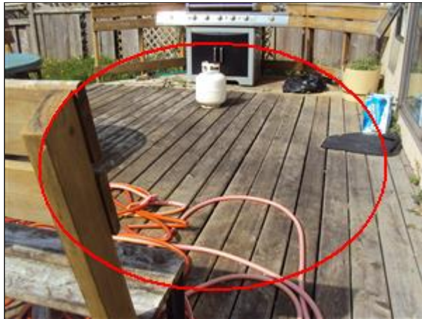
2.4 Picture 2 Repair & Stain Deck
