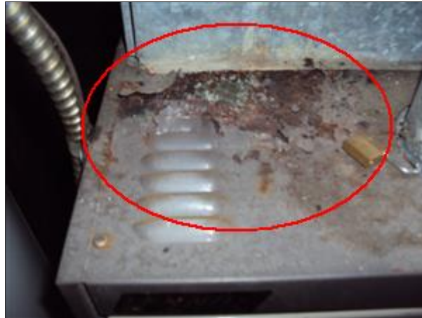
8.0 Picture 5 Corrosion
