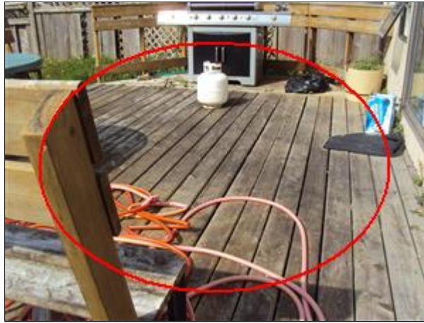
2.4 Picture 2 Repair &amp; Stain Deck
