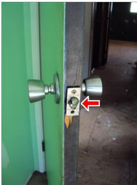
4.5 Picture 3 Broken Mechanism
