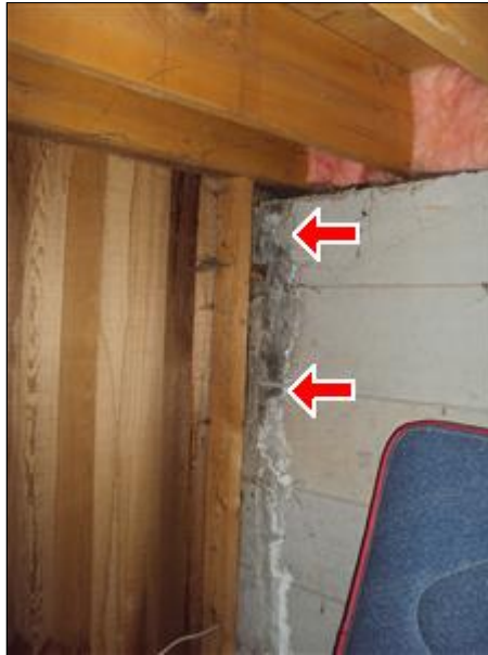
4.1 Picture 6 Efflorescence
