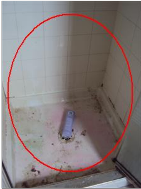
6.1 Picture 3 Clean & Seal Grout
