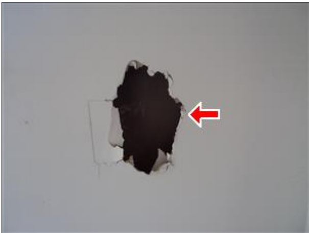
4.1 Picture 2 Interior Walls
