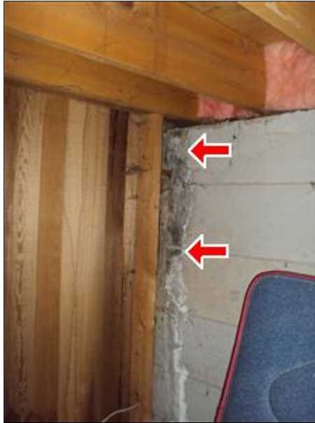
4.1 Picture 6 Efflorescence
