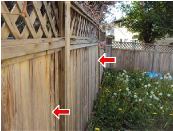
2.6 Picture 2 Perimeter Fencing
