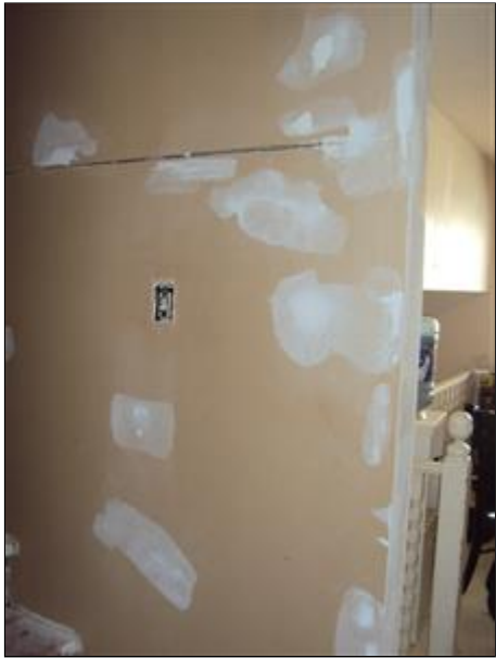
4.1 Picture 1 Interior Walls
