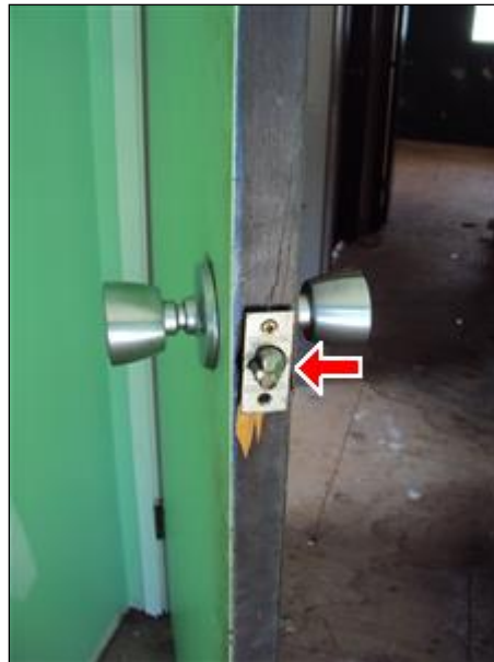
4.5 Picture 3 Broken Mechanism
