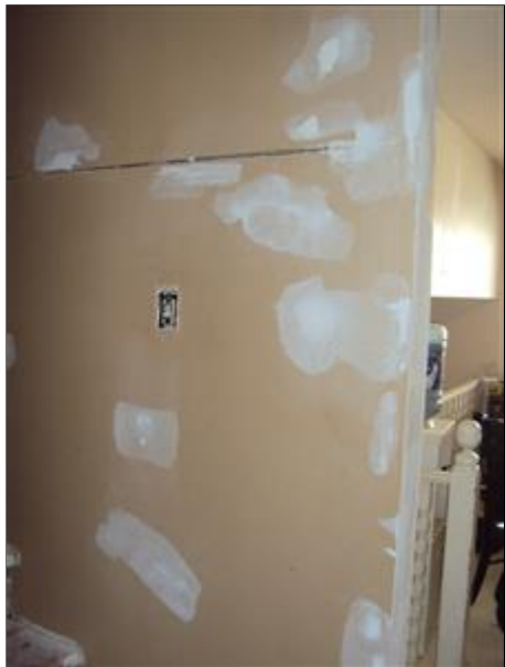
4.1 Picture 1 Interior Walls
