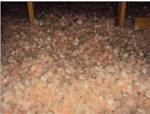
9.0 Picture 2 Blown In Insulation
