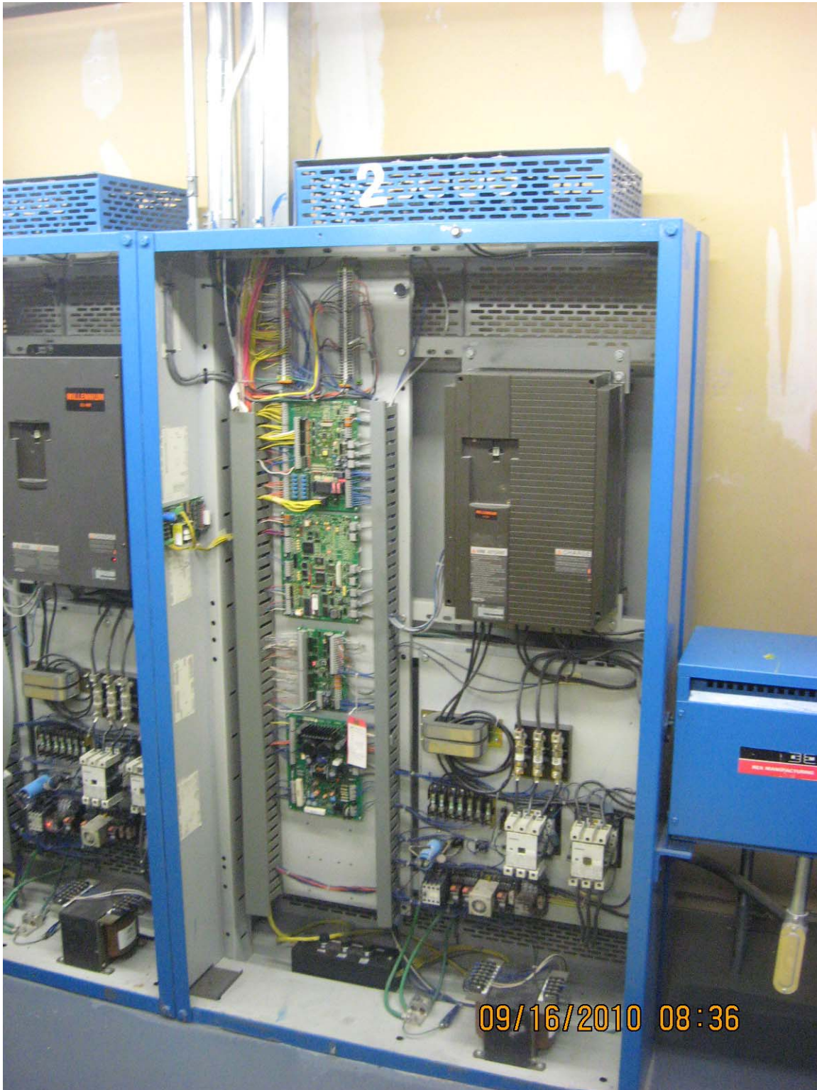
Photo 1 – Elevator Controller
