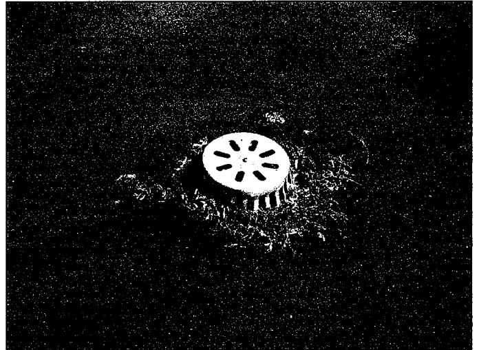
Photo #24- Debris present at perimeter of drain.
