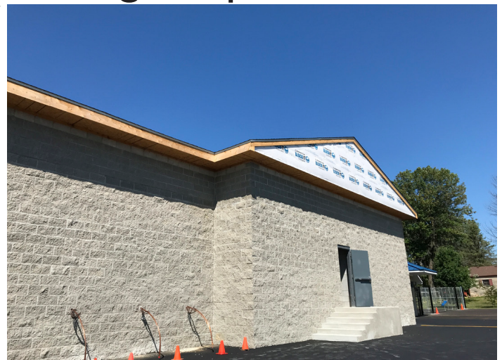
Construction for the new locker room is currently underway. Many athletes were excited about the news.
