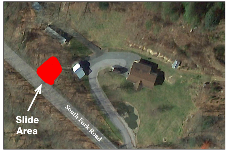
The above enhanced Google Earth view shows the Kuykendall home and garage in relation to the land slide on South Fork Road.
