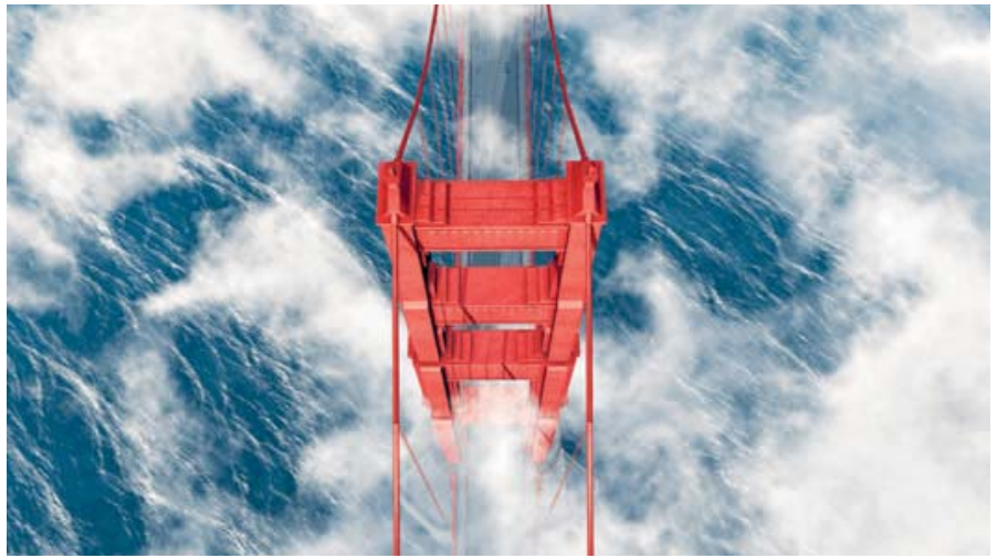
Golden Gate Bridge in San Francisco. iStock
