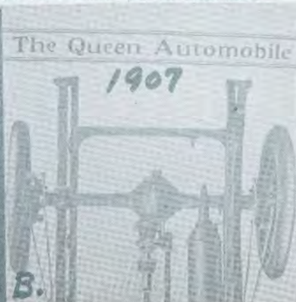
A. 17" drop center wheel (wire) B. Queen rear axle
