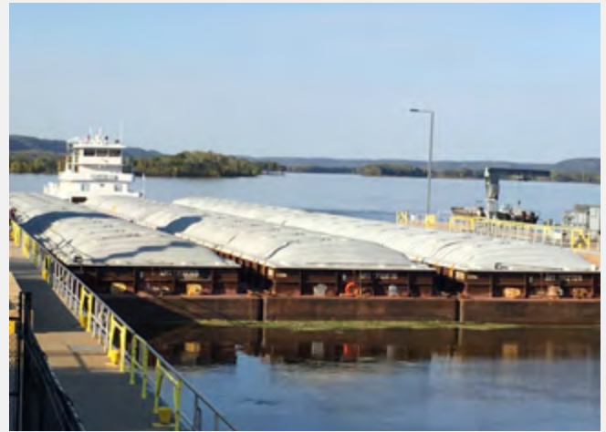
Barge Flotilla Lock and Dam
