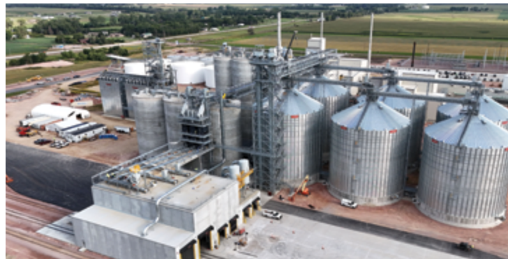
Modern rail and truck receiving infrastructure at High Plains Processing will ensure efficient grain movement and reliable delivery to domestic and international markets.
