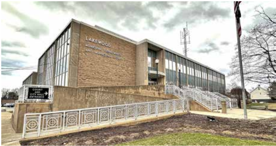
City Hall designed in the 50s, built in the 60s has been a solid performer for decades. Unfortunately time flies, and things change, and the building has not kept up with the times and technology.
