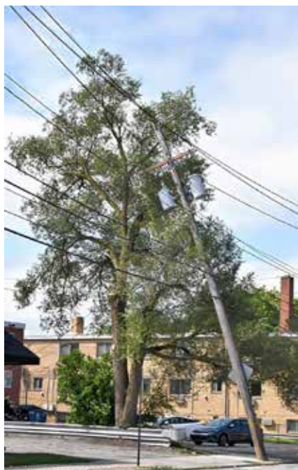
Not just Lakewood's trees took hits, many telephone poles.
