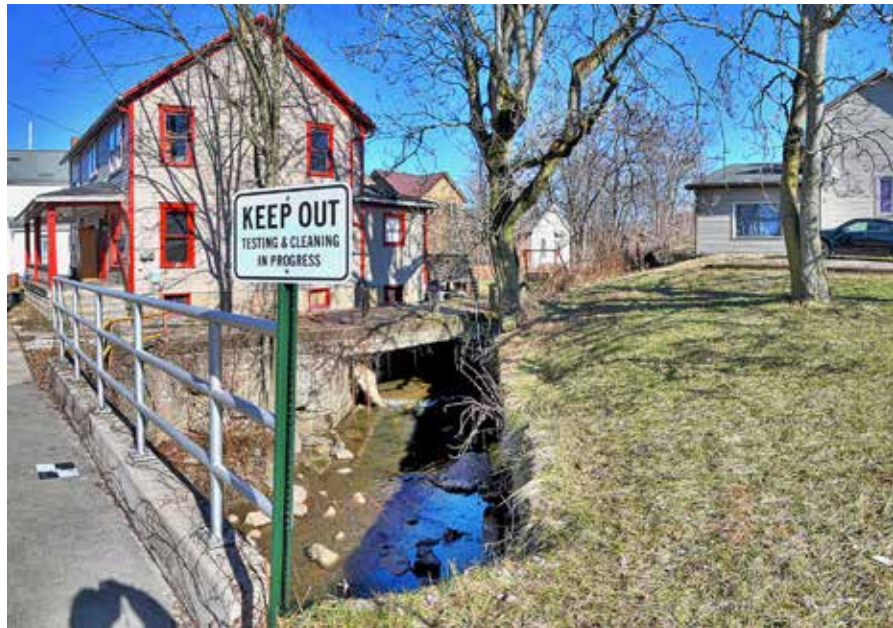
You can see the creek still flowing under the property. This is common throughout East Palestine.
