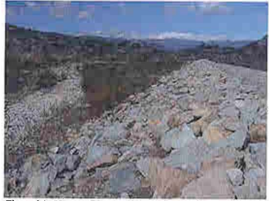
Figure 34. Ventura River Casitas Springs looking north 9.5 miles below Matilija Dam. 2-25-07
