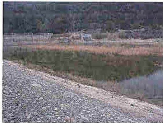
Figure 18. Robles Diversion stilling basin looking northwest 2.25 miles below Matilija Dam. 2-08-07
