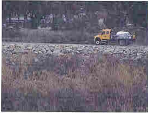
Figure 33. Ventura River Casitas Springs levee looking southeast 9.0 miles below Matilija Dam. 2-08-07
