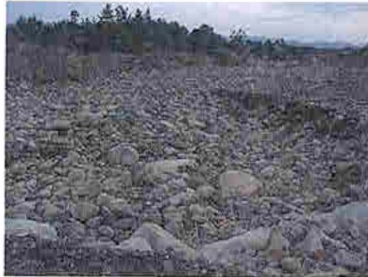
Figure 22. Ventura River (east channel) looking downstream from Robles Diversion timber cut-off wall. 2-08-07
