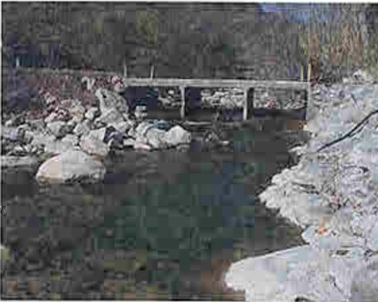
Figure 15. Camino Cielo Crossing looking north 0.75 miles below Matilija Dam. 2-23-07
