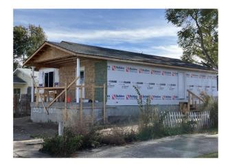
This week This week the shingles have been placed on the roof, locking doors have been added, and the first window was installed.
