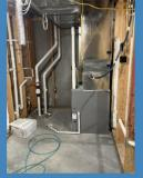
This week the furnace and ducting was installed and the sewer lift pump is plumbed into the drain lines. The bathtub was installed in the lower bathroom, and sink wall of the kitchen is plumbed with hot and cold water, drain lines and electrical work is also done!
