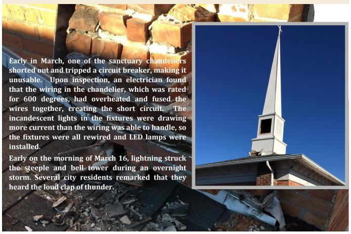
Church staff first became aware of a problem when internet access was unavailable. A Comcast technician responded promptly and restored internet access after finding that an outdoor ground splitter had been melted by the lightning strike. Steeple damage is still clearly visible from the south parking lot, and masonry damage to the tower is visible from North Street.
